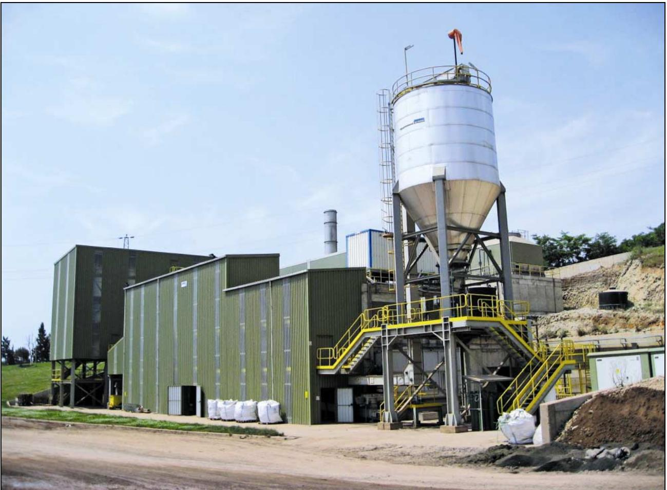
In many cases, a large part of the energy released as waste gas from the rotary kiln in cement production goes to waste. The NUH Cimento works in Hereke, Turkey, is one of the most outstanding examples of innovative ANDRITZ technology, where the sewage sludge is dried using waste heat from cement production and the dried granulate then used as auxiliary fuel to generate heat for cement production.
