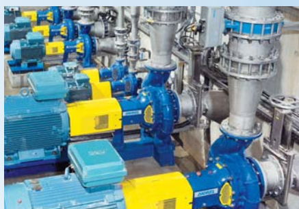
◀ Process pumps for conveying water and suspensions in different industries such as pulp and paper
