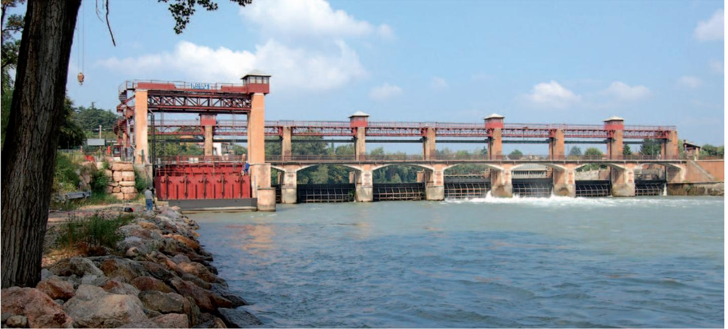
In Verona's district of Chievo a dam and adjacent ship lock were built in the 19th century on the Adige River to establish the Camuzzoni canal. The abandoned ship lock downstream of the Chievo dam owned by Consorzio Canale Camuzzoni was modified to harvest the unused hydropower potential of the abandoned lock without compromising its flood discharge capabilities.
