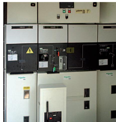
The electrical equipment setup is completed by step-up transformers, high-voltage switchgear, and station service equipment. At the Chievo dam all these systems have been placed in two operation buildings located in close vicinity to the module. The power and control cables of the turbine generator units are run inside of the module gallery and are collectively routed to the landside generator switchgear using a flexible cable chain, cable trays and conduits.
