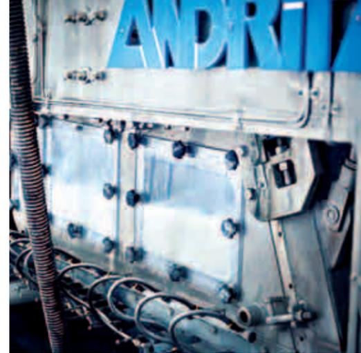
▲ To produce KROMOPAK, the conventional vacuum formers on PM3 had to be replaced by a fourdrinier wet section. Adding the new *PrimeForm HB* hybrid former on the filler layer enabled the correct level of dewatering and improved formation.
