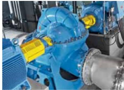
▲ The ANDRITZ headbox pump for PM2 operates at an impressive 92% efficiency.
